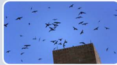
Knutti Hall Boiler House
